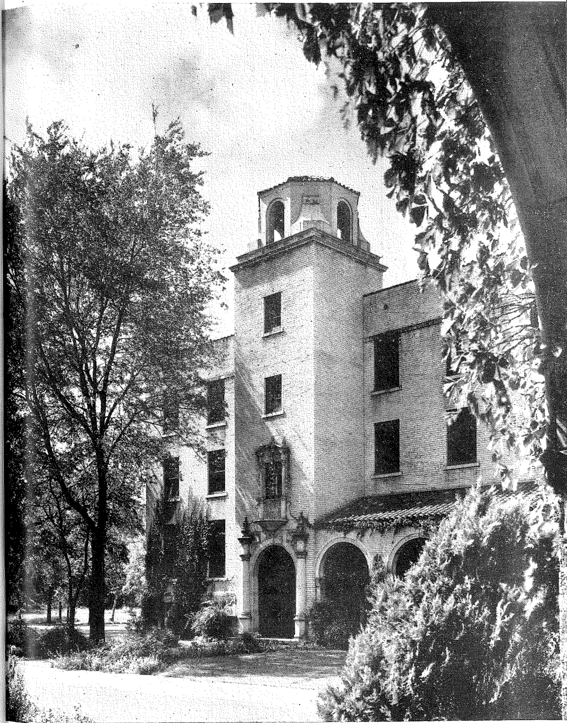
STEARNS HALL, DORMITORY FOR SINGLE MEN
